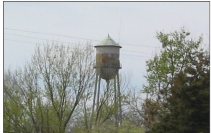
Elevated water tower in Beggs, OK
